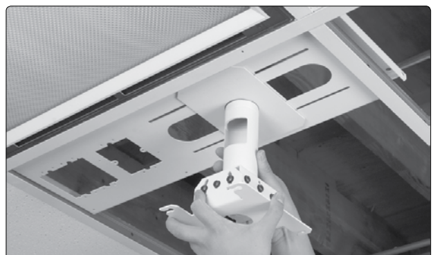
2d Screw the adjuster plate onto the PMP
